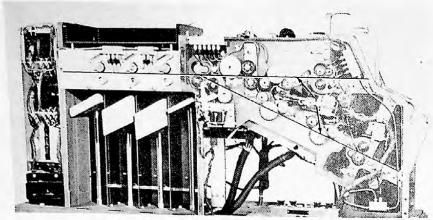
Figure 48. Card Feed Unit — Type 77 Collator
